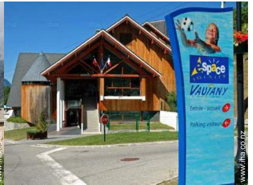
Covered swimming pool
